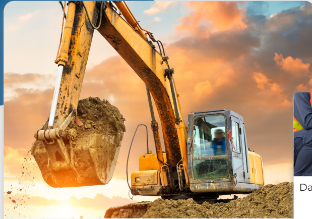
Ground Disturbance Level 2
